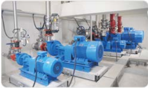
PUMP equipment (The maximum horsepower is 1100KW per unit)
