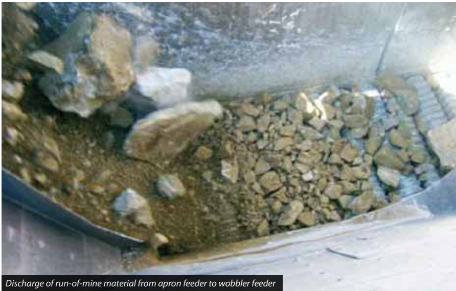
Discharge of run-of-mine material from apron feeder to wobbler feeder
