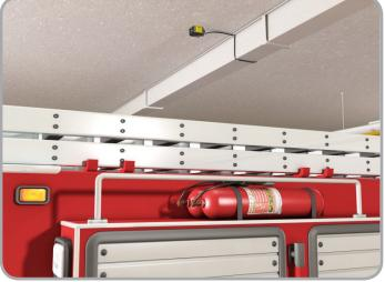
R-GAGE™ retroreflective radar sensors installed over vehicle stalls in a fire station detect vehicle presence and record departure and arrival times for fire trucks
