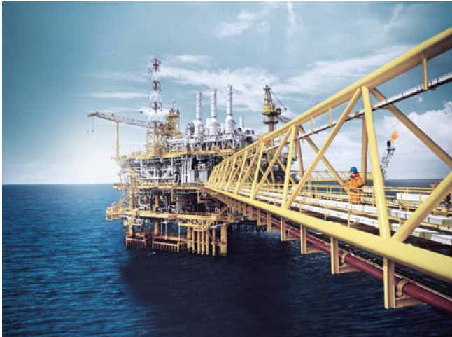
Flare gas measurement on offshore platforms...
