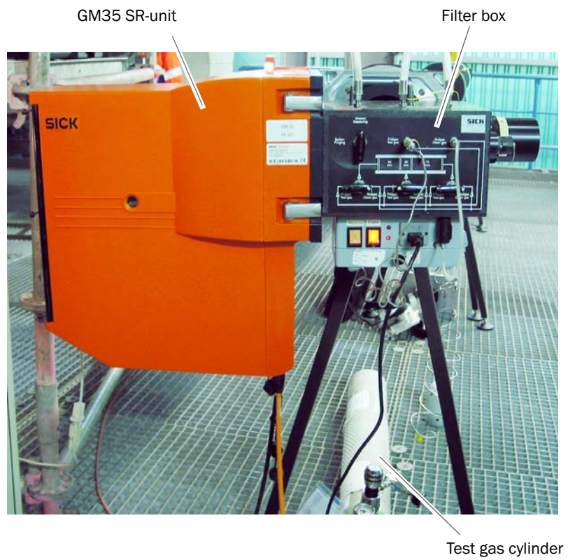
Fig. 65: Installing the filter box
