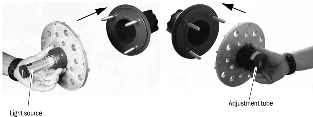
Fig. 7: Aligning the flange using an optical adjustment device
