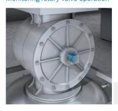
Rotary valves are small components in an aluminum plant but they play an important role in the flow of materials and in guaranteeing uninterrupted production. Typical applications for rotary valves include discharging dust from silos, bunkers, hopper gates, and transfer points in conveying systems. The axial movement of the rotary valves can be monitored using the DFS60 incremental encoder.
