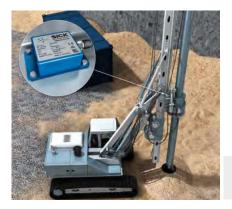
The foundation for successful drilling is accurate positioning and adjustment of the drilling machine. To do so, the TMM88 inclination sensor determines the x- and y-coordinates. High accuracy over the entire measuring range,
